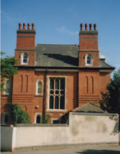
Fine house compromised by 'repairs' to boundary wall
